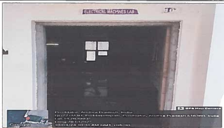
Electrical Machines Lab(Front View)
