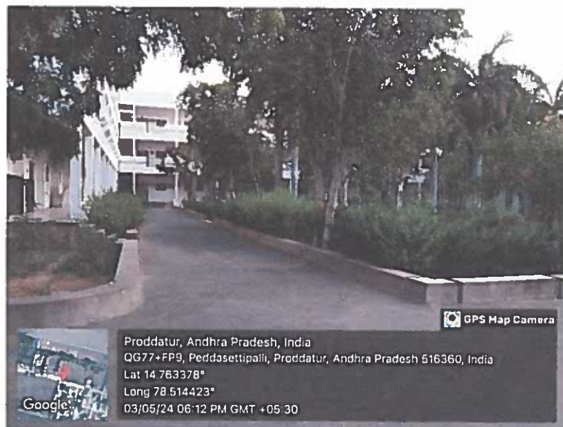
College Building S-Block
